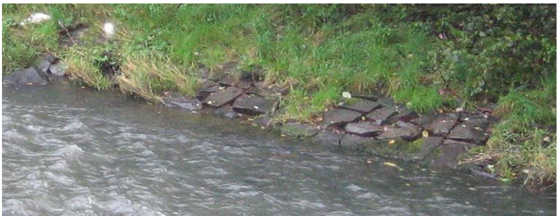
Figure 4: Border reinforcements along the shores of the river Bigge at sample site B3
