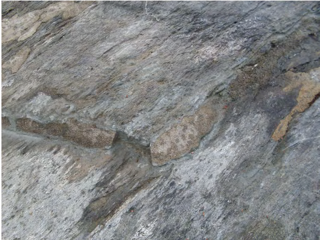
Figure 69. Area at the Ausevik outcrop in which previous cement-based mortar filling and sealing of less cohesive areas had to undergo maintenance work with the resealing of the cement/parent rock interface.
