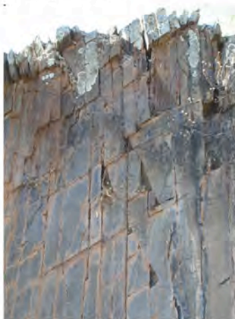
Non-engraved area of Rock 1 with with great profusion of fractures and fissures. Note also minor toppling.
