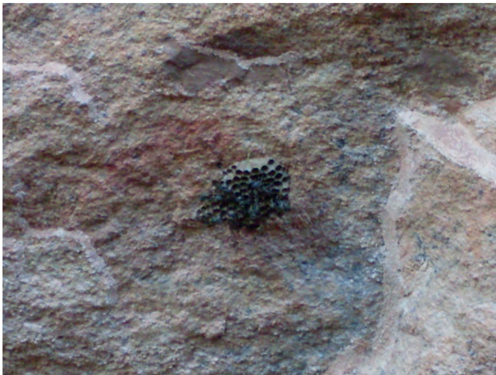
Figure 82. Biodeterioration threat in the form of a wasp nest.
