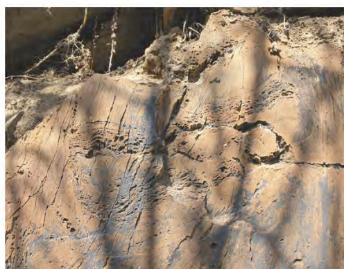
Weakness area due to aveolization, gaping and fracturing.
