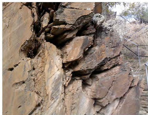
Fractures, disconnected blocks and exfoliation near the engraved panel.
