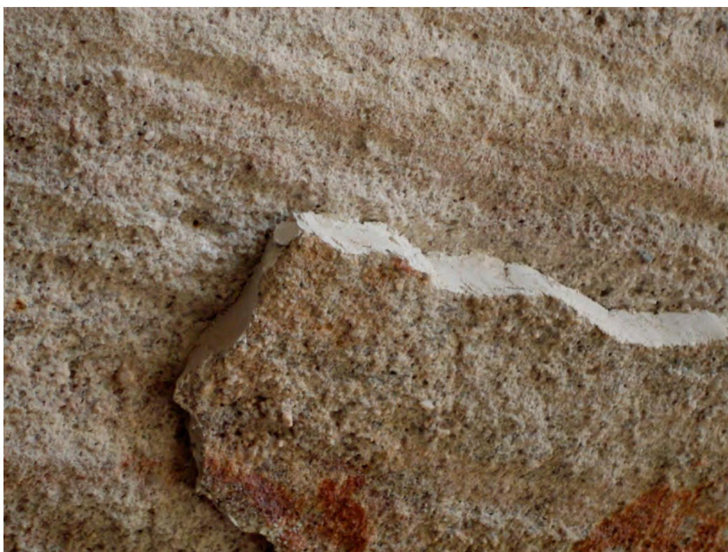
Figure 84. Sealed part of a panel that was in risk of detachment.
