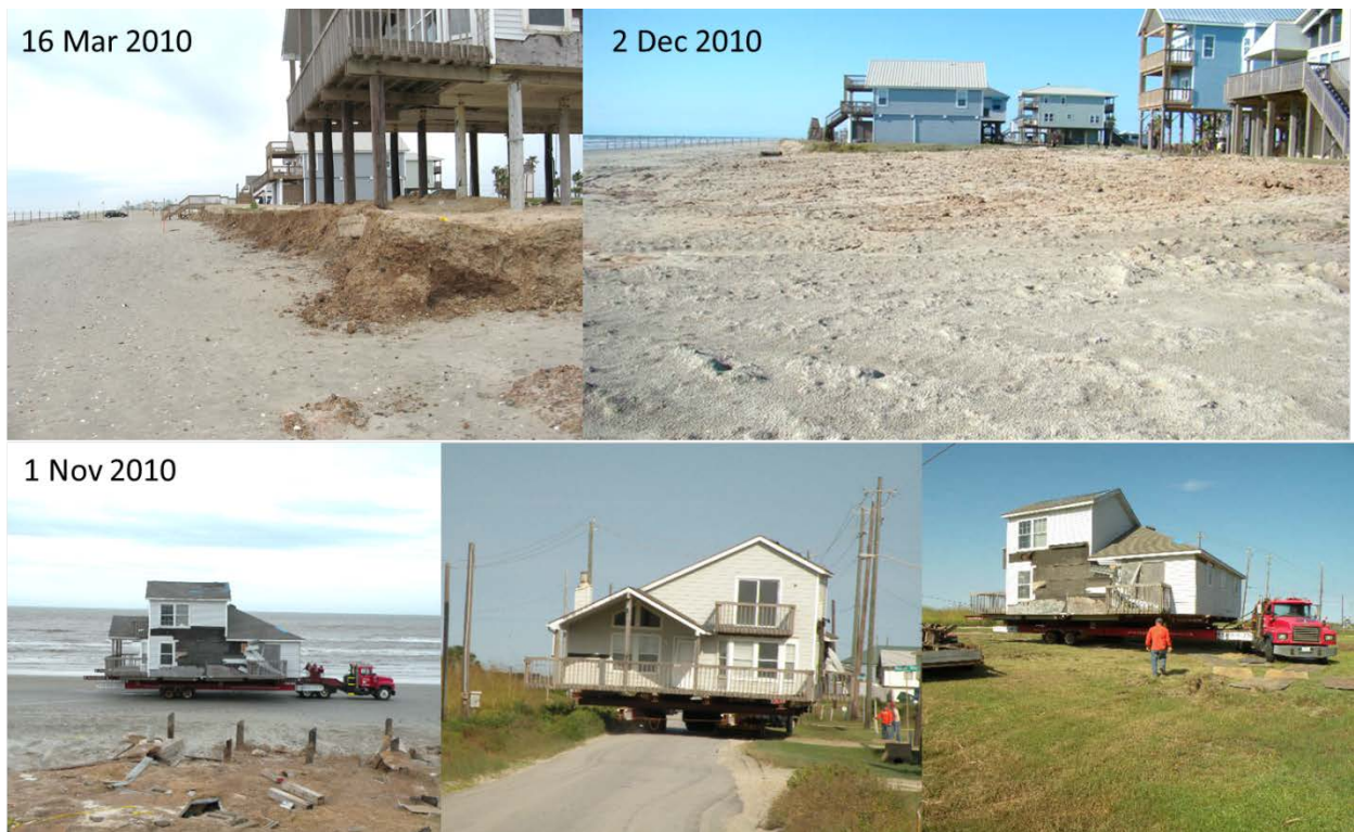
Figure 17. Example of house relocation under the Texas Open Beach Act. The house location was within the public beach easement at Sunny Beach, West Galveston Island (top left) and was relocated further
