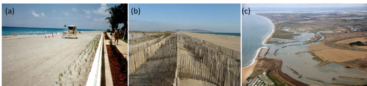
Figure 4. Examples of soft engineering schemes: (a) beach nourishment in Palm Beach, Florida, USA (photo: L.S. Esteves); (b) dune restoration in Lido de Sete, French Mediterranean coast (photo: Jon J. Williams); and (c) managed realignment in Wallasea Island, UK (photo: John Akerman).
