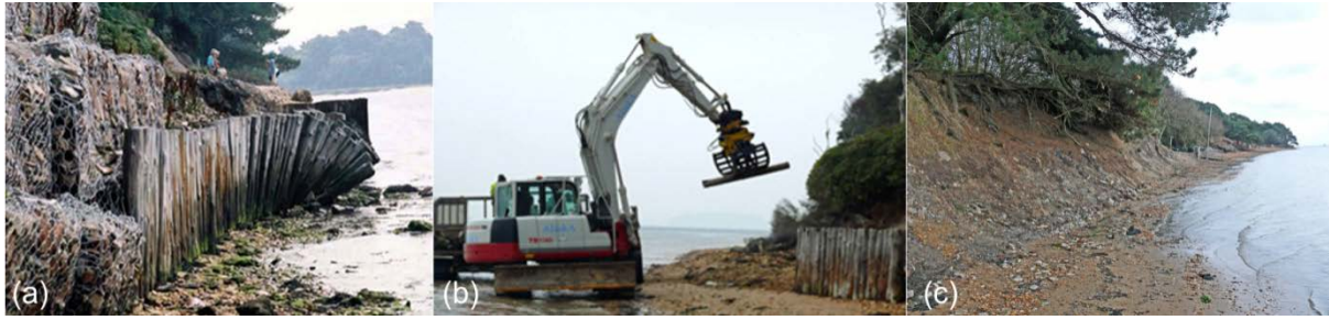
Figure 23. Failing defences in Brownsea Island (a) were removed in 2011 (b) and by early 2013 the shoreline showed an appearance similar to the time before sea defences were built (c).
