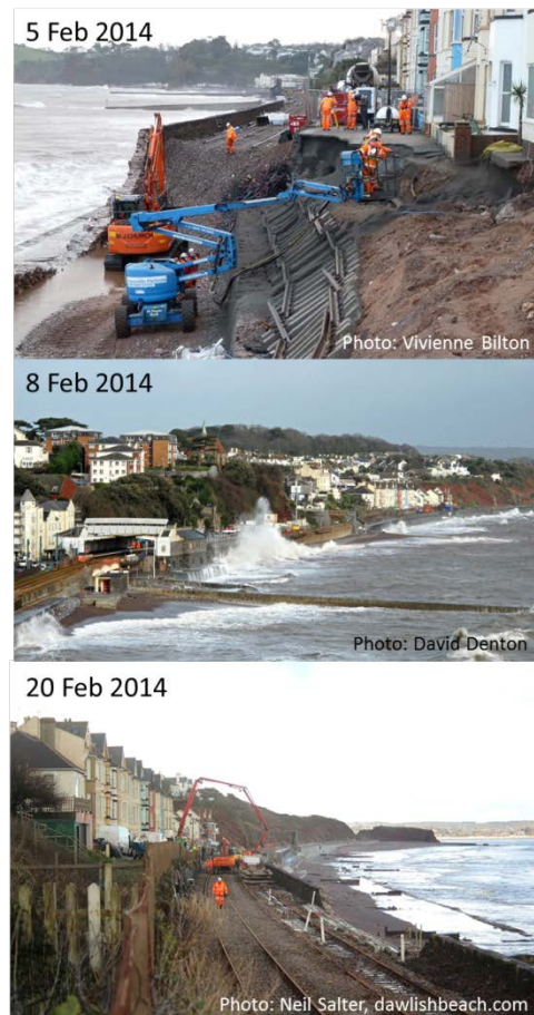
Figure 2. A long spell of stormy weather has caused major impact at the coast of southwest England in January and February 2014. Coastal defences have been overwhelmed at Dawlish where the railway line collapsed cutting rail links to Cornwall and west Devon. A number of houses located next to the rail line were affected and the seawall and groynes were greatly damaged.
