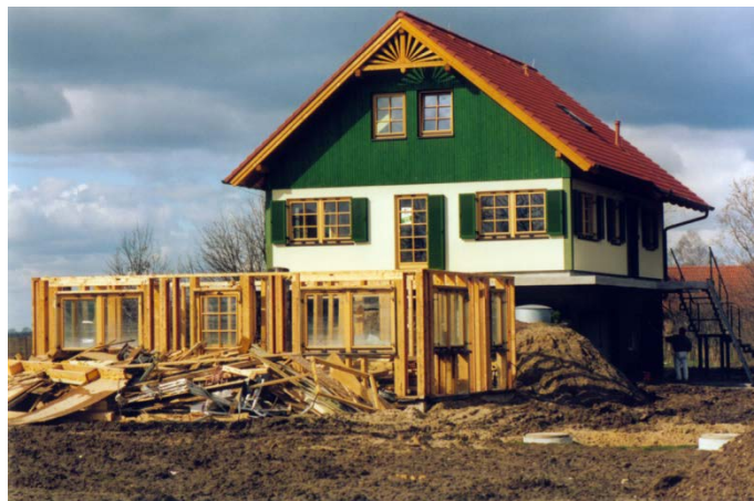
Figure 1. Adaptation can take many forms. This house had just been built (in Ziltendorfer Niederung, the floodplain of the River Oder in Germany) when it was flooded in the summer of 1997. Afterwards the owner decided to re-build the house in a slightly retreated position and on an elevated level, so the ‘ground floor’ would be less prone to flooding. The photo shows the original position of the house and how it looks after ‘redevelopment’. Photo courtesy of Baerbel Koppe, AQUADOT Engineering Consultants, Hamburg).
