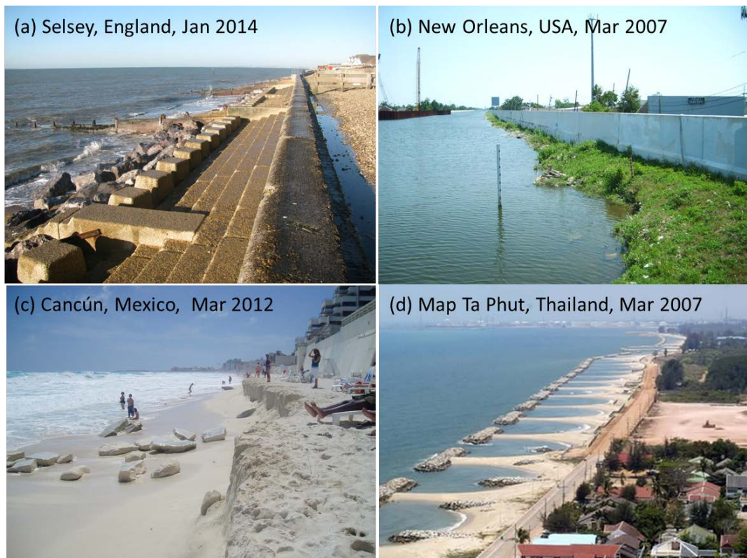
Figure 3. Hard engineering structures are shaping coasts and rivers worldwide, causing natural habitat loss and favouring development in hazard-prone areas. (a) Storms have greatly reduced the beach fronting coastal defences in Selsey, an area also prone to flooding (photo: L.S. Esteves). (b) Flood defence along the Mississippi river close to where a breach occurred during hurricane Katrina causing devastating flooding (photo: L.S. Esteves). (c) Cancún is a narrow barrier beach densely occupied by hotels and subjected to intense erosion due to hurricanes impacts; hotels survival depends on beach nourishment and hard engineering beach nourishment (photo courtesy of Grupo de Ingeniería de Costas y Puertos del Instituto de Ingeniería, UNAM). (d) Map Ta Phut suffers critical coastal problems due to the engineering works that support the large industrial park in the country (photo courtesy of Andy Coburn, Western Carolina University).
