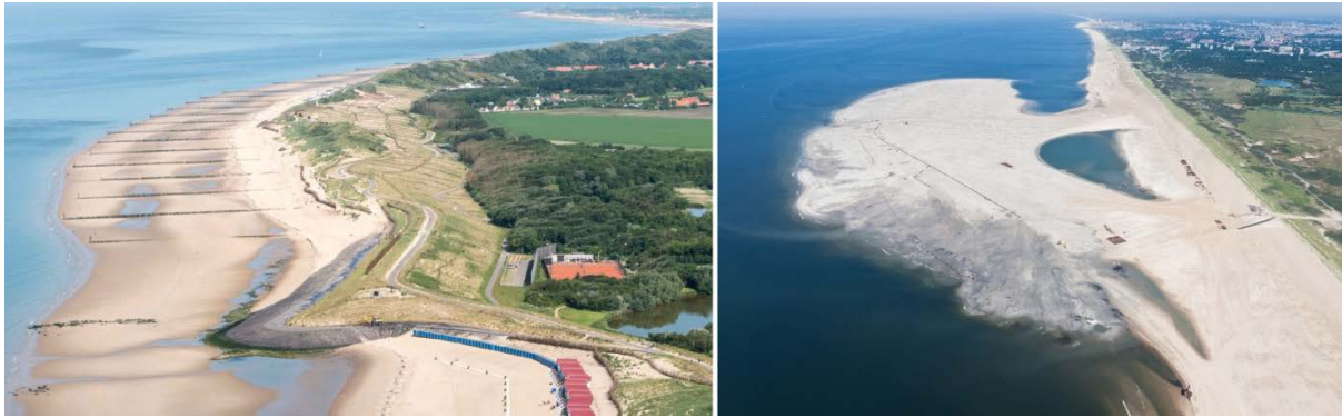
Figure 19. Beach nourishments and dike-dune reinforcements (left) as part of the Weak Links project have improved both flood safety and spatial quality at Nolle-Westduin near Vlissingen, SW Delta. The Sand Motor project (in the right during construction phase in 2011) involves a large sand nourishment along the eroding coast south of The Hague. Photos: courtesy of Rijkswaterstaat.
