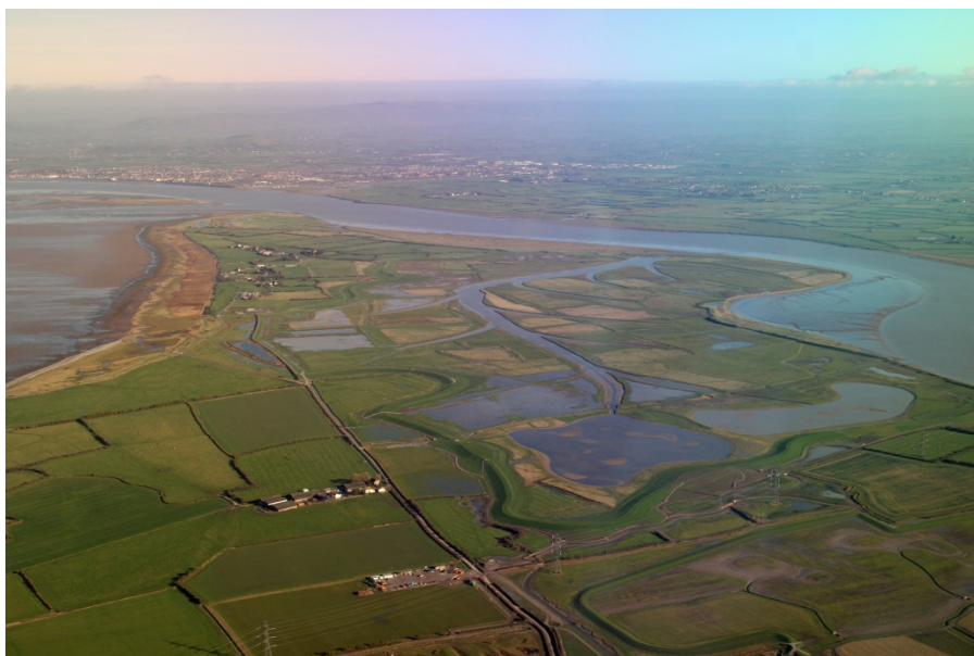
Figure 31. Steart Coastal Management Project in the River Parrett is due to be opened in autumn 2014. This scheme has two objectives: to provide compensatory habitat and to improve flood defences for the local community. Note that the breach has not yet occurred at the time of the photo, the water seen within the scheme is freshwater due to a particularly wet winter. Photo courtesy of the Environment Agency.
