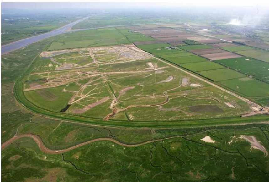
Figure 30. Hesketh Out Marsh West in the Ribble Estuary during the construction phase. The scheme covers about 168 ha and was opened in 2008 with the principal objective being to create compensatory intertidal habitat. Photo courtesy of the RSPB.
