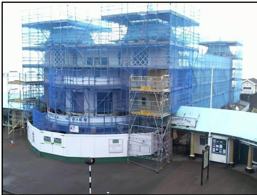
Figure 2: Penarth pier pavilion undergoing rehabilitation in 2012. Picture: Chris Wyatt
