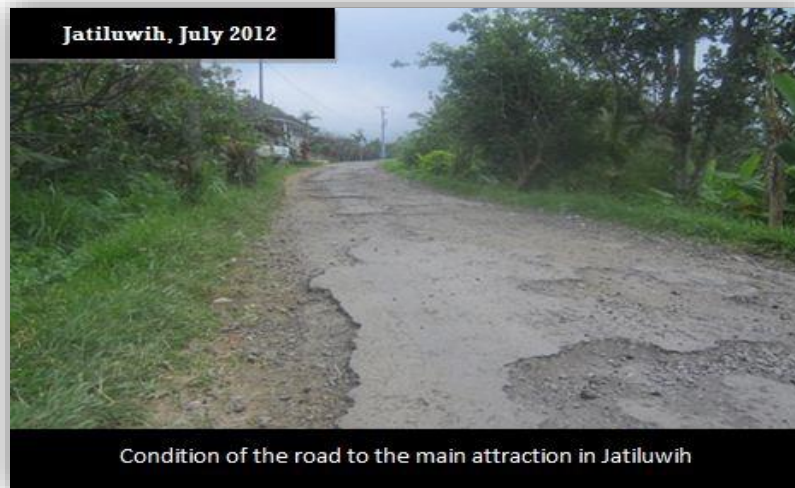
Figure 6.5: Condition of Roads in Jatiluwih village
