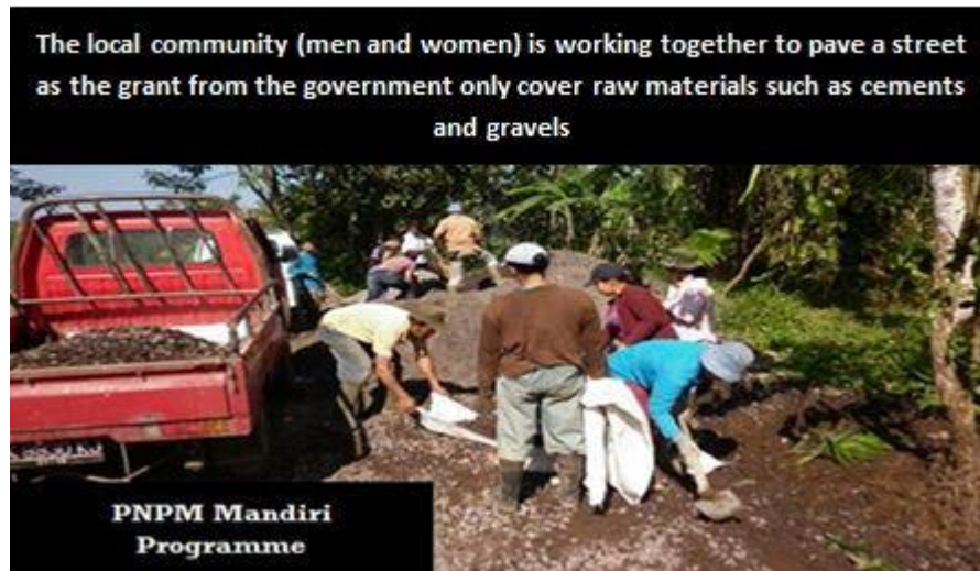
Figure 6.2: PNPM programme for renovating a street in Jatiluwih village.
