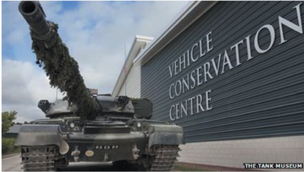
Figure 3: Building of the new conservation facility at The Tank Museum. Image courtesy of The Tank Museum.
