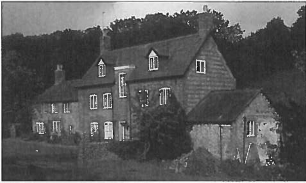
Figure 1: Woolcombe farmhouse south elevation, 1997, showing (to the right) the single storey byre with white painted wall-scar that denotes the area that was shared with the demolished bottling plant (Bournemouth University BU ).
