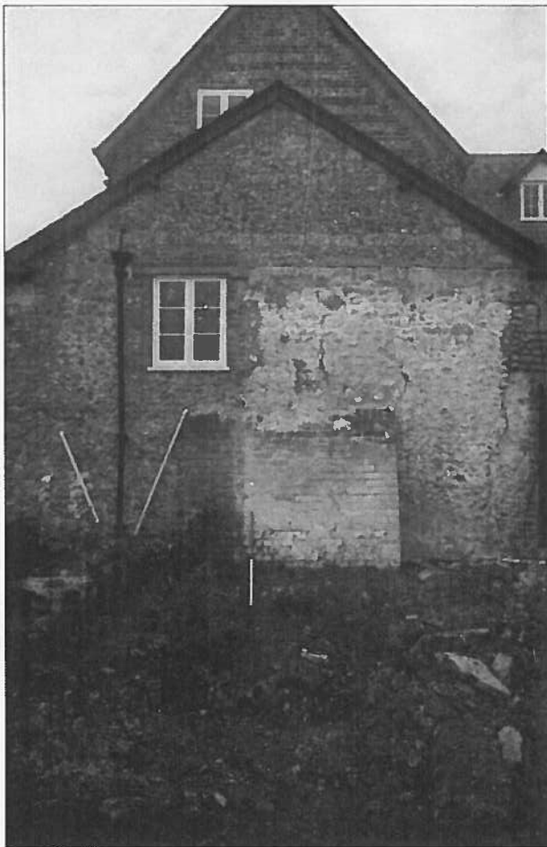
Figure 9: The east elevation of Woolcombe farmhouse in 1997 showing the ground floor byre wall. The white-painted area to the right of the downpipe and window represents the area adjoined by the former bottling plant. This part of the wall seems to have been made good and it is supported by a brick buttress (Bournemouth University).
