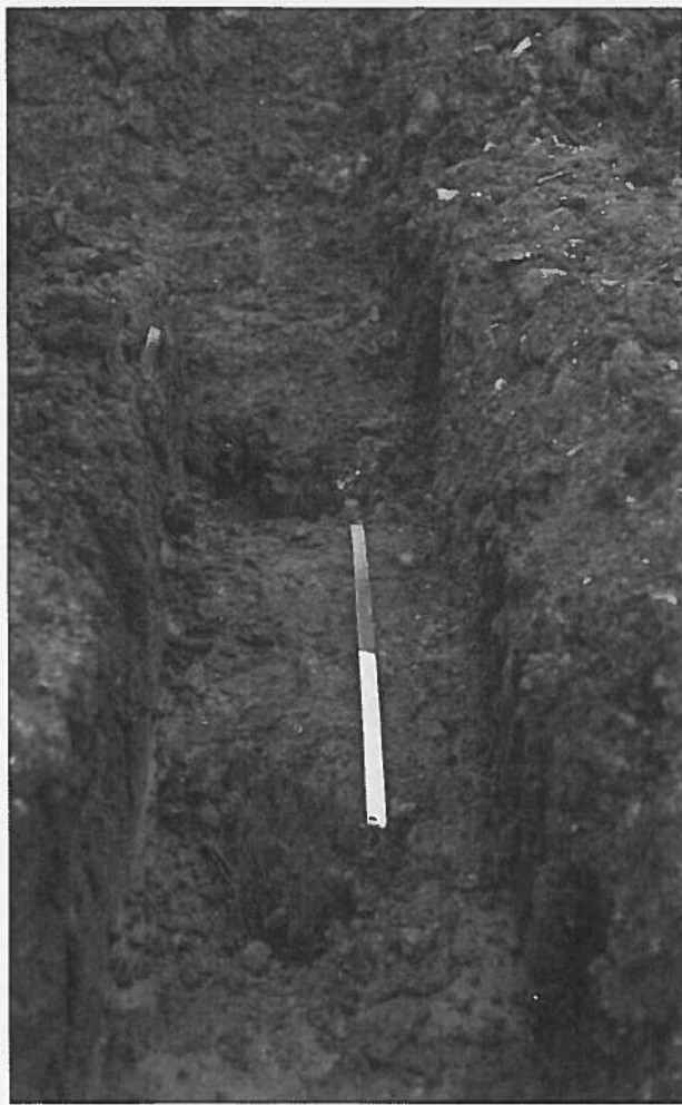
Figure 13: The bottling plant site (1997). Two of the remnant hardwood stumps (Figure 13 nos 2 and 3) can be seen within the new foundation trench (Bournemouth University).
