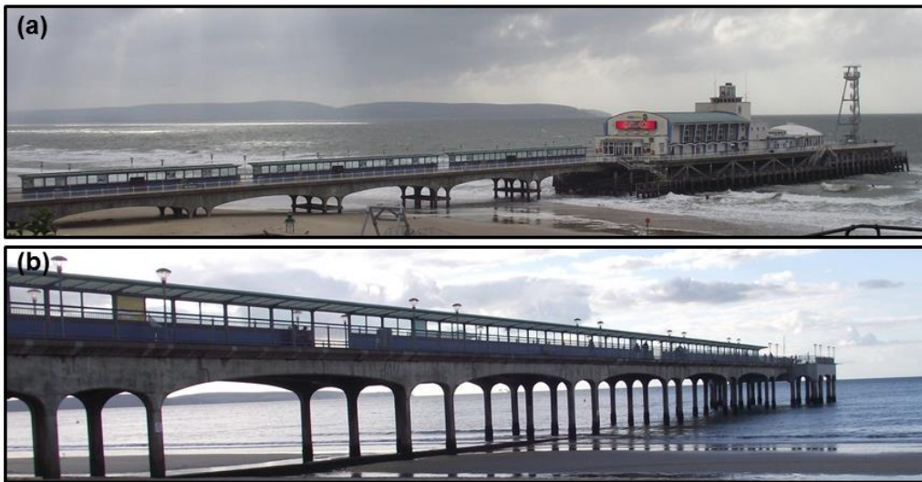
Figure A2.1: Images of a) Bournemouth Pier and b) Boscombe Pier to illustrate variation in structural complexity.
