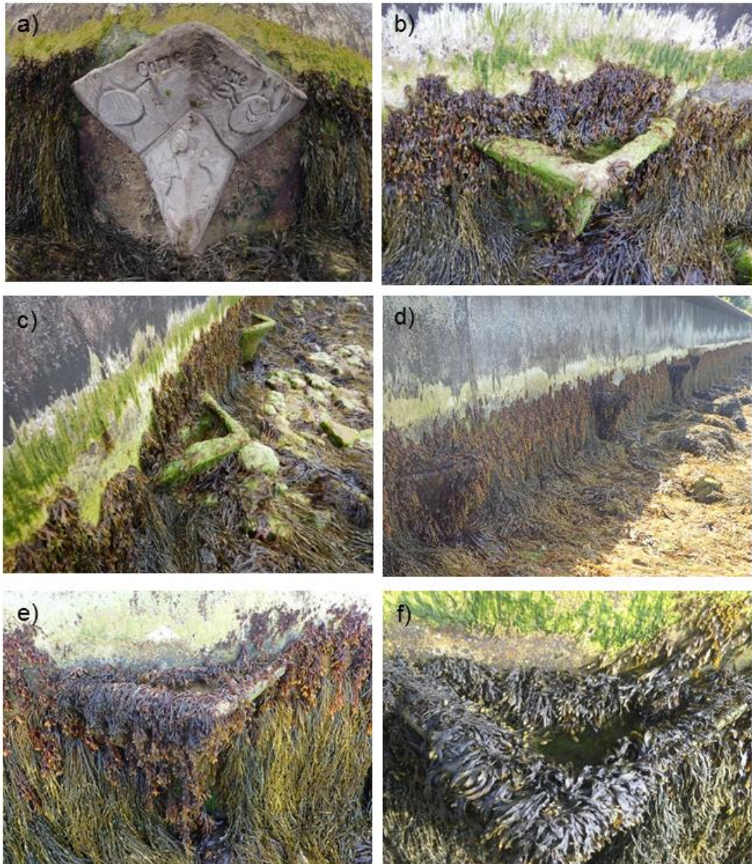
Figure 7.1 Images of the Vertipools; a) Vertipool and cleared area immediately after installation in 2013, showing detail of exterior design, b) Vertipool after 2 years, c) and d) positioning of Vertipools on seawall, e) and f) Vertipools after 3 years.
