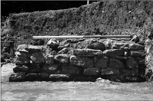
Figure 1: East face of the excavated wall section showing the sandstone construction. The scale is 1 m in length.
