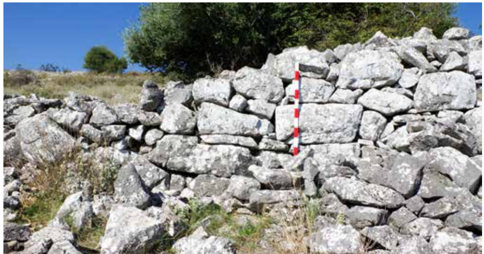
Fig. 15. Outer face of wall between Tower 7 and Tower 8 , looking towards the west. Photograph by S. Chandrasekaran.
