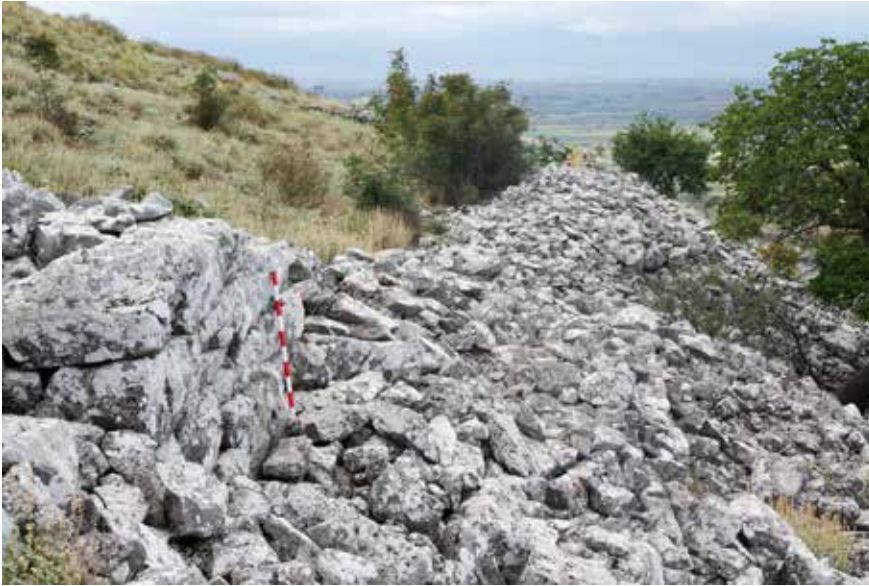
Fig. 33. Nearly obliterated section of Phase 2B fortification wall, as seen from Tower 21 , looking towards the south-west. Photograph by S. Chandrasekaran.
