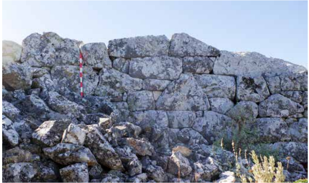
Fig. 14. Outer face of south-west descending wall, below Postern 4 , looking towards the east. Photograph by S. Chandrasekaran.
