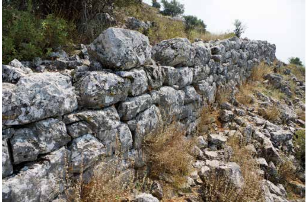
Fig. 35. West end of diateichisma, looking towards the east. Photograph by R. Rönnlund.
