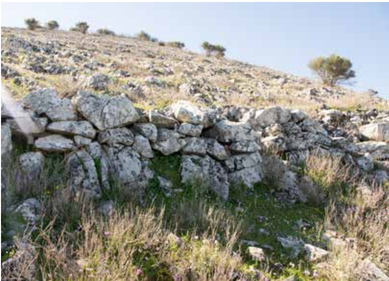
Fig. 28. Detail of masonry in retaining wall of the North road , looking towards the south-south-east. Photograph by R. Rönnlund.
