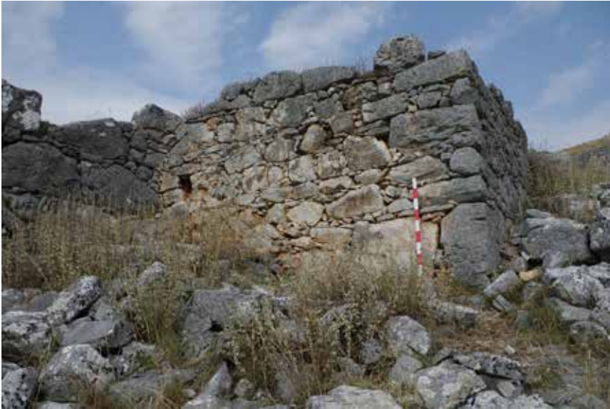
Fig. 52. South-east face of Tower 2 , looking north-west. Photograph by R. Rönnlund.
