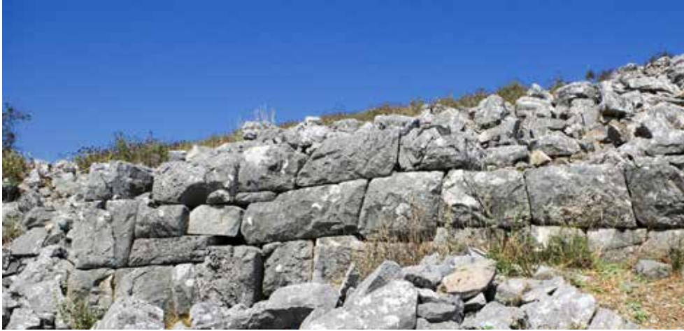
Fig. 37. South side of Tower 3 , showing the irregular trapezoidal masonry. Photograph by R. Rönnlund.
