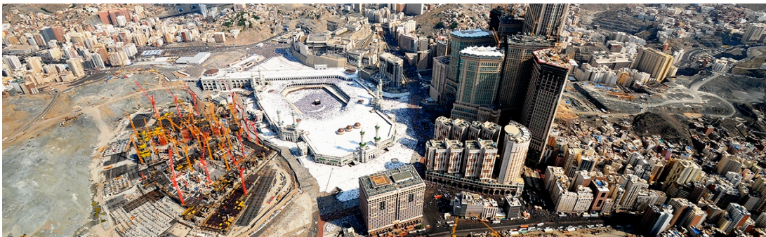
Figure 1-5: Jabal Omar Project Under Construction (Hill n.d.)
