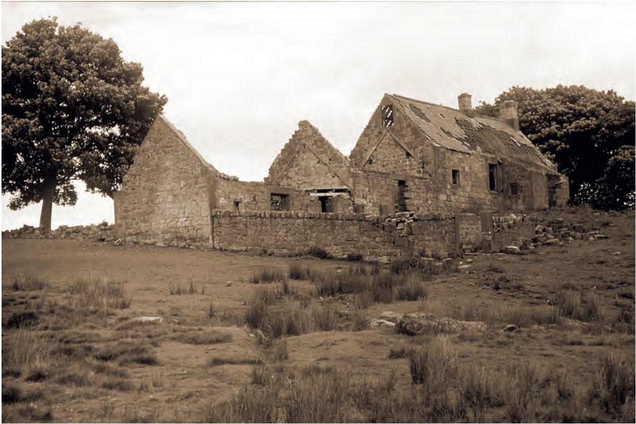
Figure 1. Blawearie shepherd's house from the west south-west, 1975. Photograph by Stan Beckensall.
