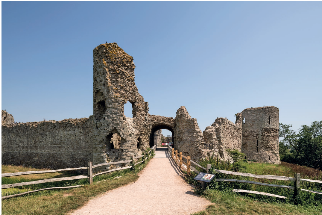
Fig. 7. Fortunately, some of the north turret of the gates survives showing Master Simon's work; unfortunately, much of the south turret does not. It is accordingly difficult to ascertain if there was a significant difference between the fabric of the upper parts of the two turrets. [DP236352] © Historic England Archive
