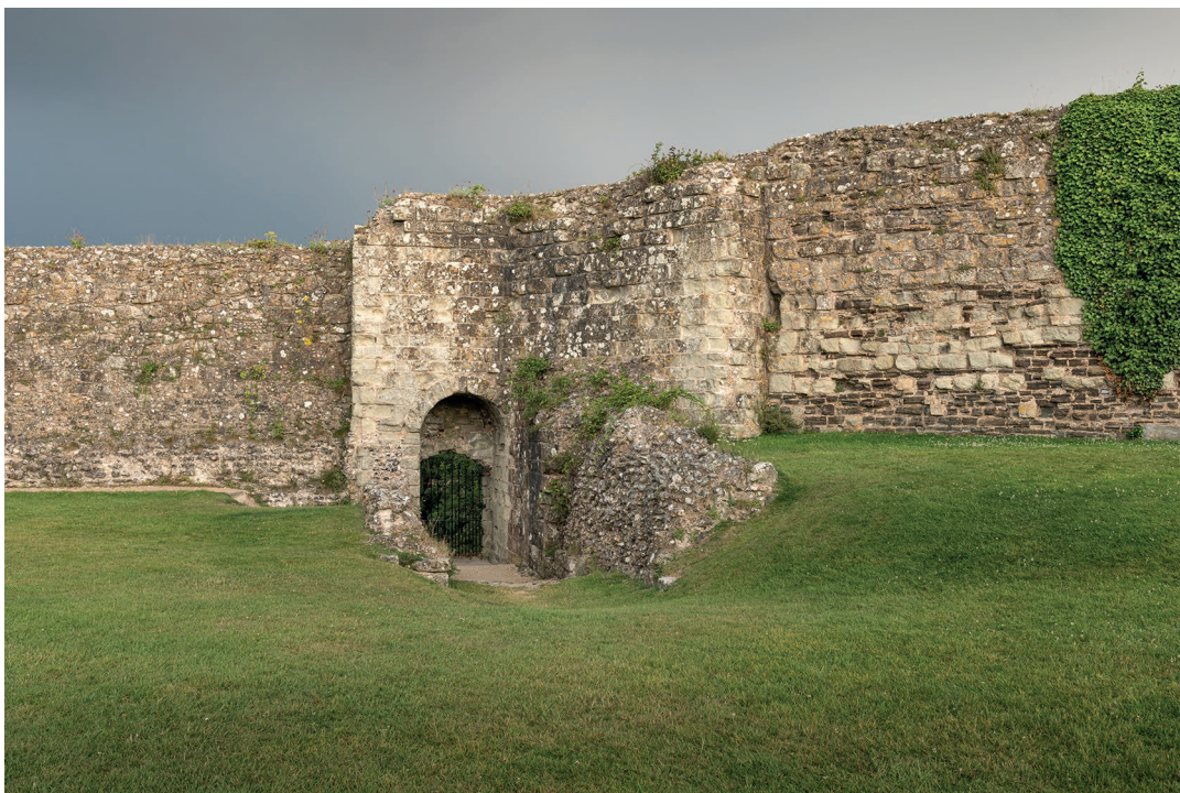
Fig. 4. There are clear joints between the postern gate and the Roman wall to the left, and the mid-13th century castle wall to the right. The wall projecting forwards may have been designed to link with the earlier earth and timber fortification. [DP236364] © Historic England Archive
