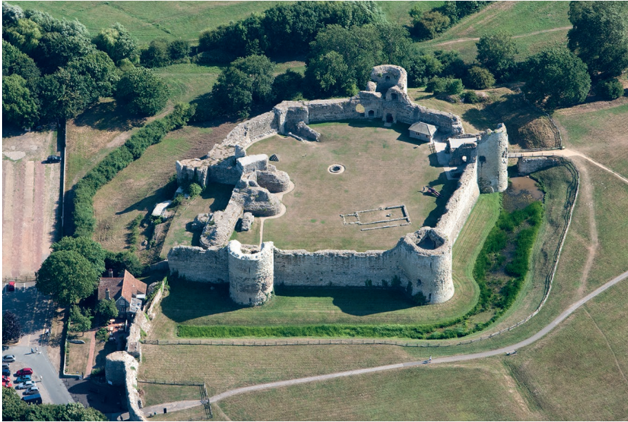
Fig. 5. The postern gate can be seen at the top left of this view with a section of Roman wall to the left of it. The medieval castle appears to have been built clockwise, beginning with its south side (top), then the main gate on the right-hand side, followed by the west and north walls. On the left-hand side, the remains of the keep and the absent, collapsed section of the east wall of the Roman fort can be seen. [26764/031] © Historic England Archive
