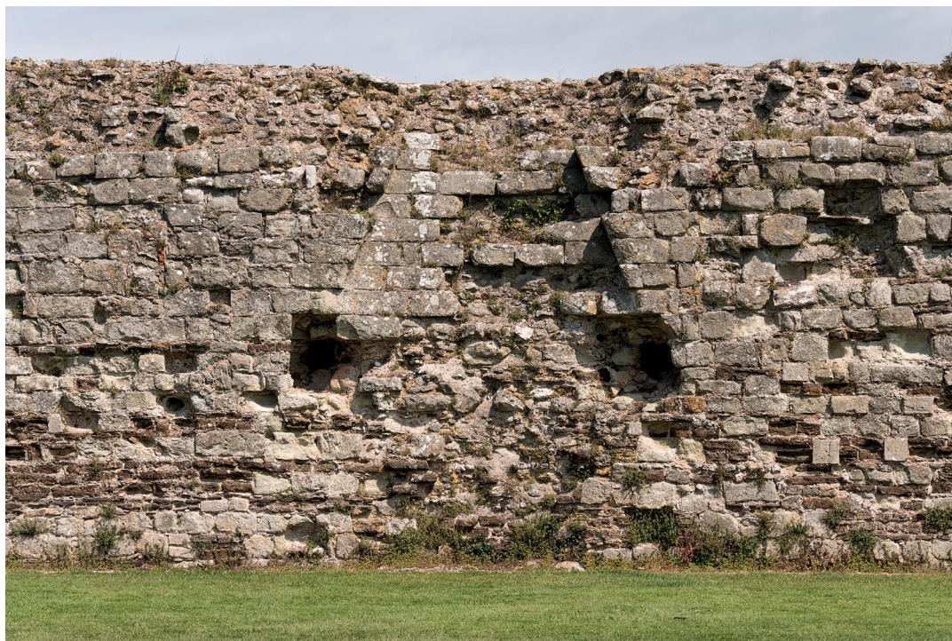
Fig. 9. One of the fireplace positions in the north wall of the medieval castle; the position of the fireplace is marked by the stonework for the back of the flue and the holes on either side where two corbels formerly supported the hood. [DP236430] © Historic England Archive
