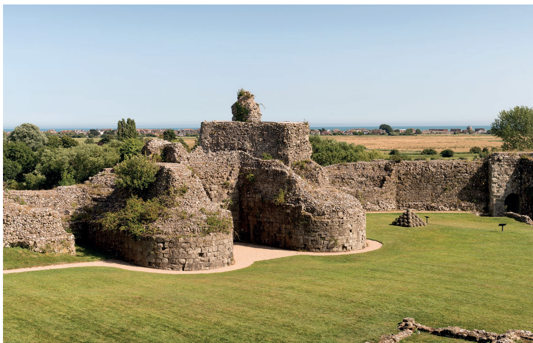
Fig. 2. The undisturbed stonework of the ground floor of the keep is in contrast to the robbed-out rubble core, surviving above. A fragment of wall that may have formed the base of the stair into the keep can be seen on the left of the photograph; to the extreme right is the postern gate, which was probably rebuilt in 1193. [DP236256] © Historic England Archive
