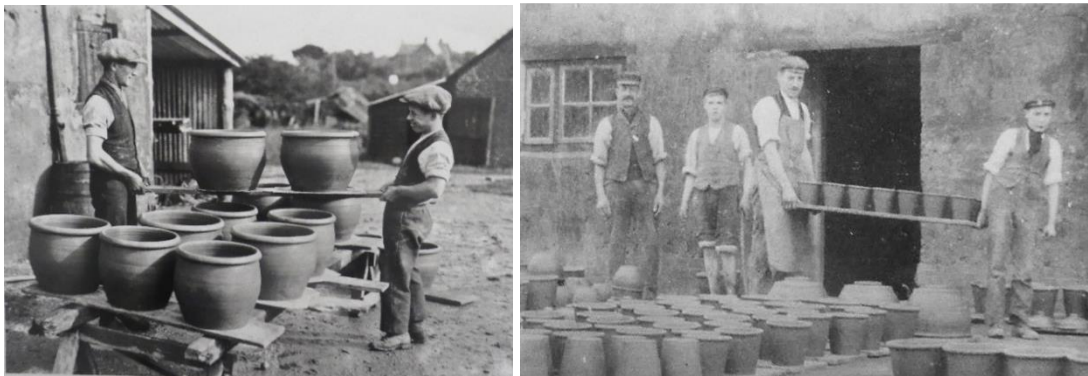
Plates 34 and 35: Wares on boards for drying at Crossroads in the early 20th century (Plate 34 from Copland-Griffiths Collection Ref. 106.12; Plate 35 MED Accession ref. WIMPH.2017.323.1; courtesy of MED)
