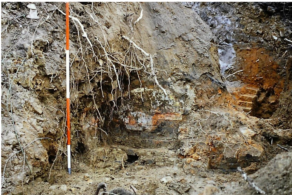
Plate 42: Splashed lead brickwork, above burnt brickwork, in the stoke shed at Black Hills, Verwood. Shown with a 2m scale; (taken from the Black Hills project archive currently held by the author)
