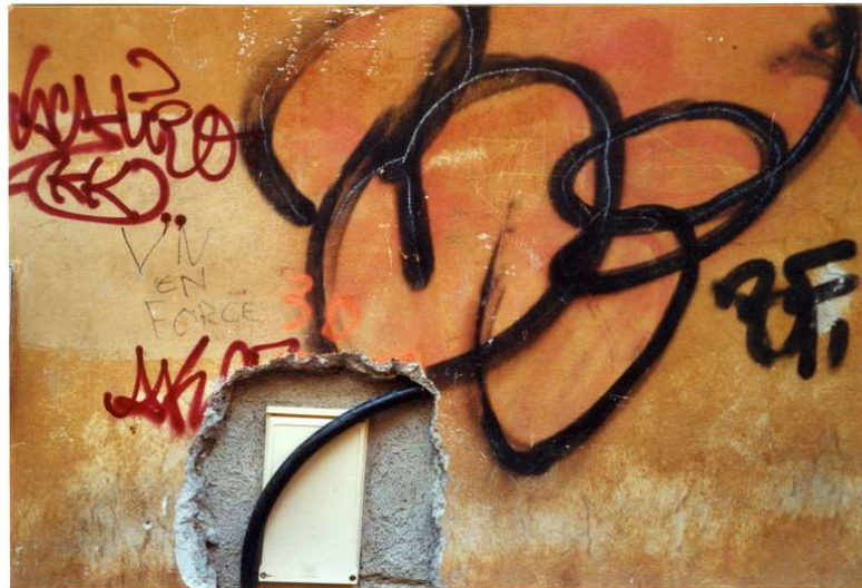
Figure 10: Nice wall #3 (hole & pipe) © Rutherford 2002
