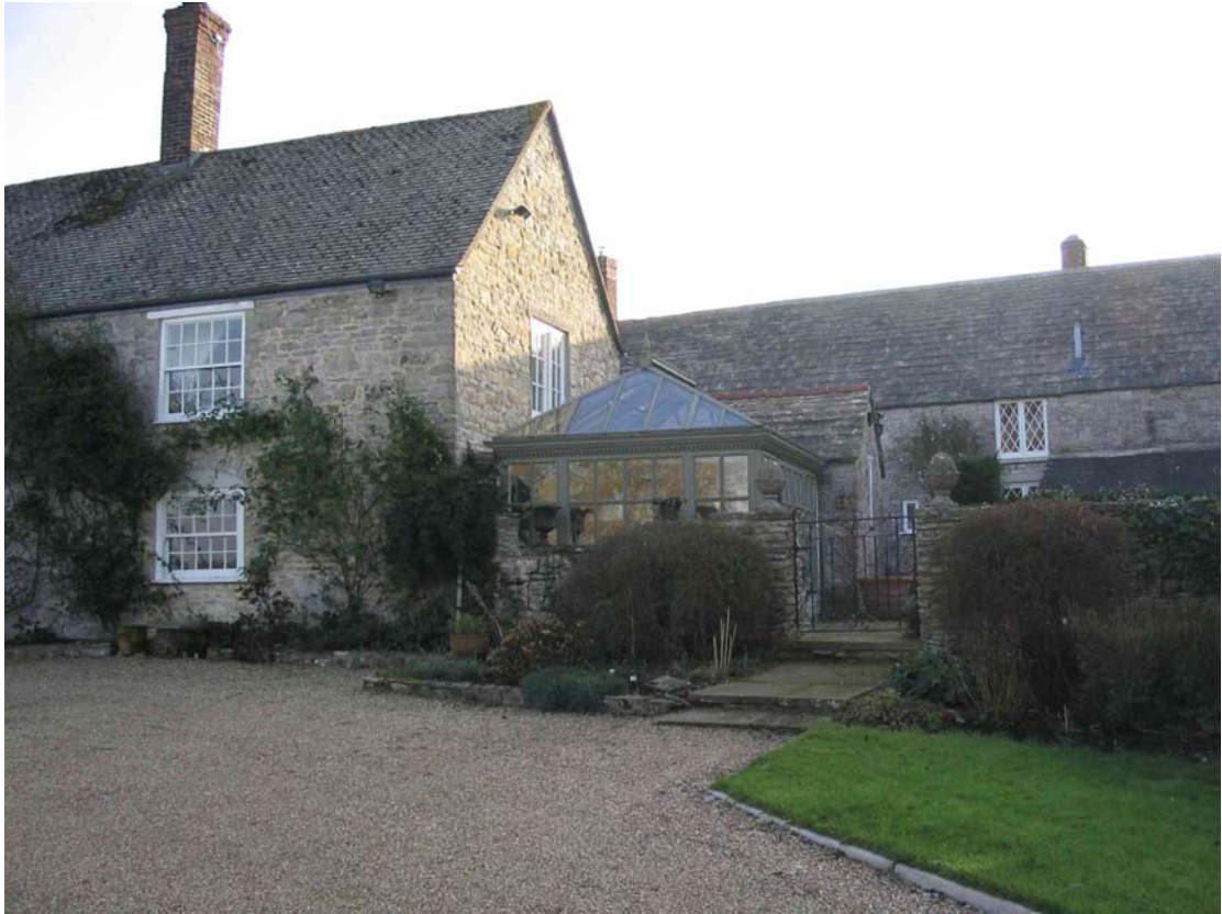
Figure 21: Photograph looking southeast . The site lies through the gate , to the east.
