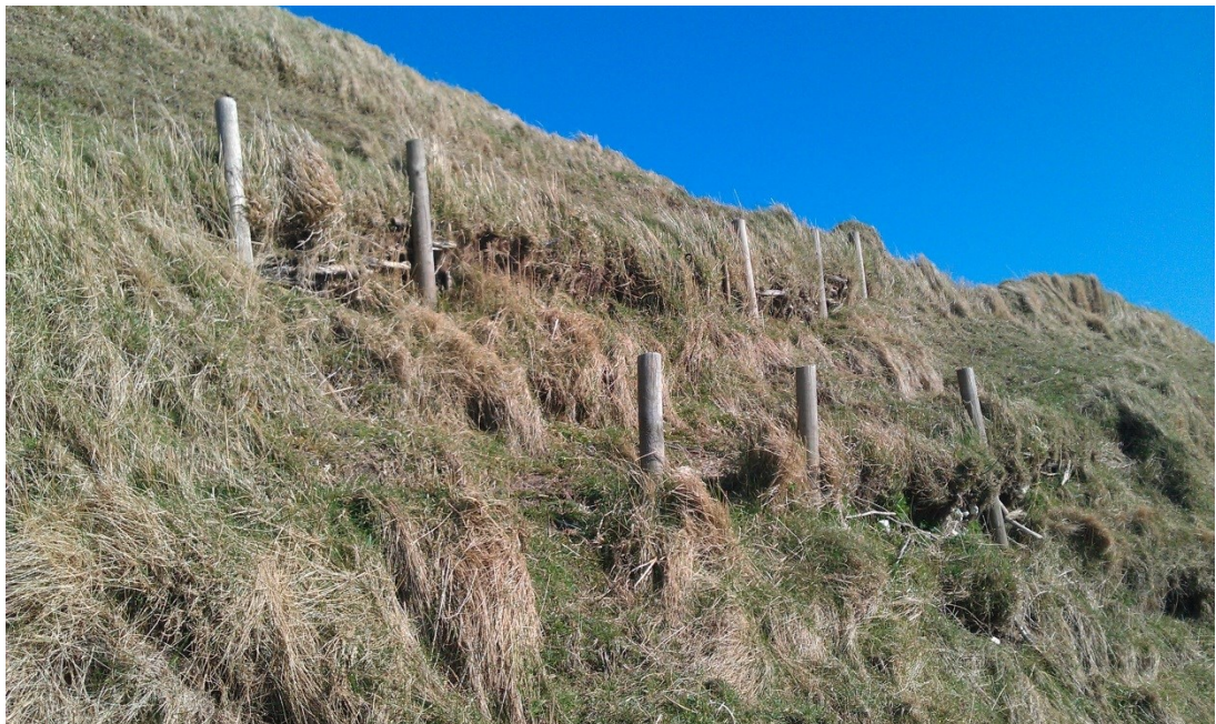
Figure 7.5: Repair works conducted on the southern ramparts of Eggardon Hillfort by the National Trust.
