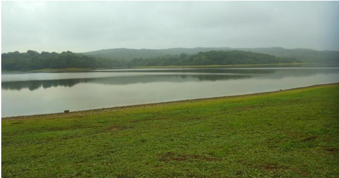
Figure 2.3 Site 3, Darwell Reservoir, October 2013.
