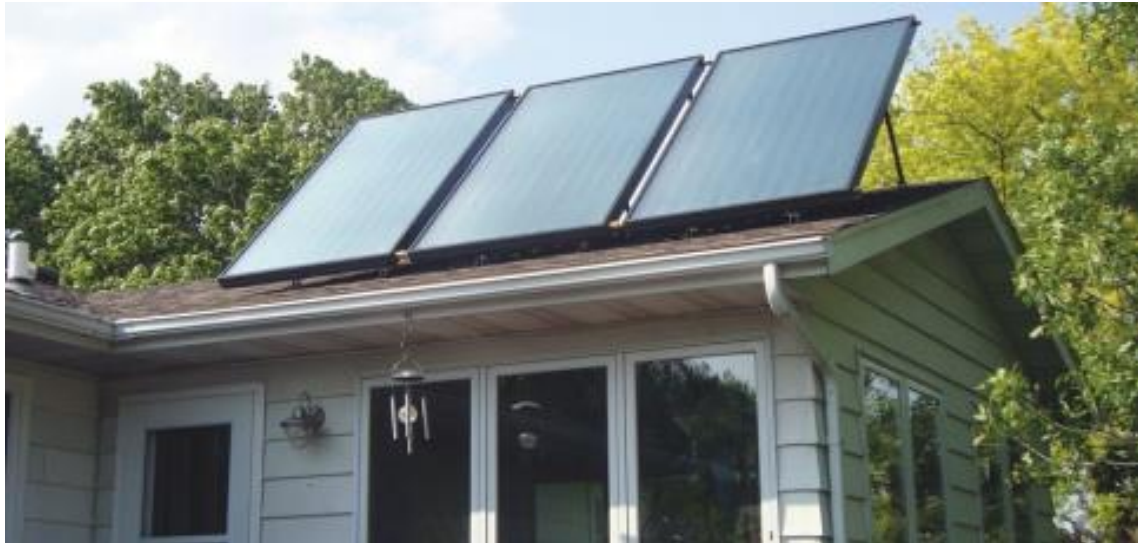
Figure 2.24: Free-standing mounted solar heat collectors on roof (Source: homepower.com)
