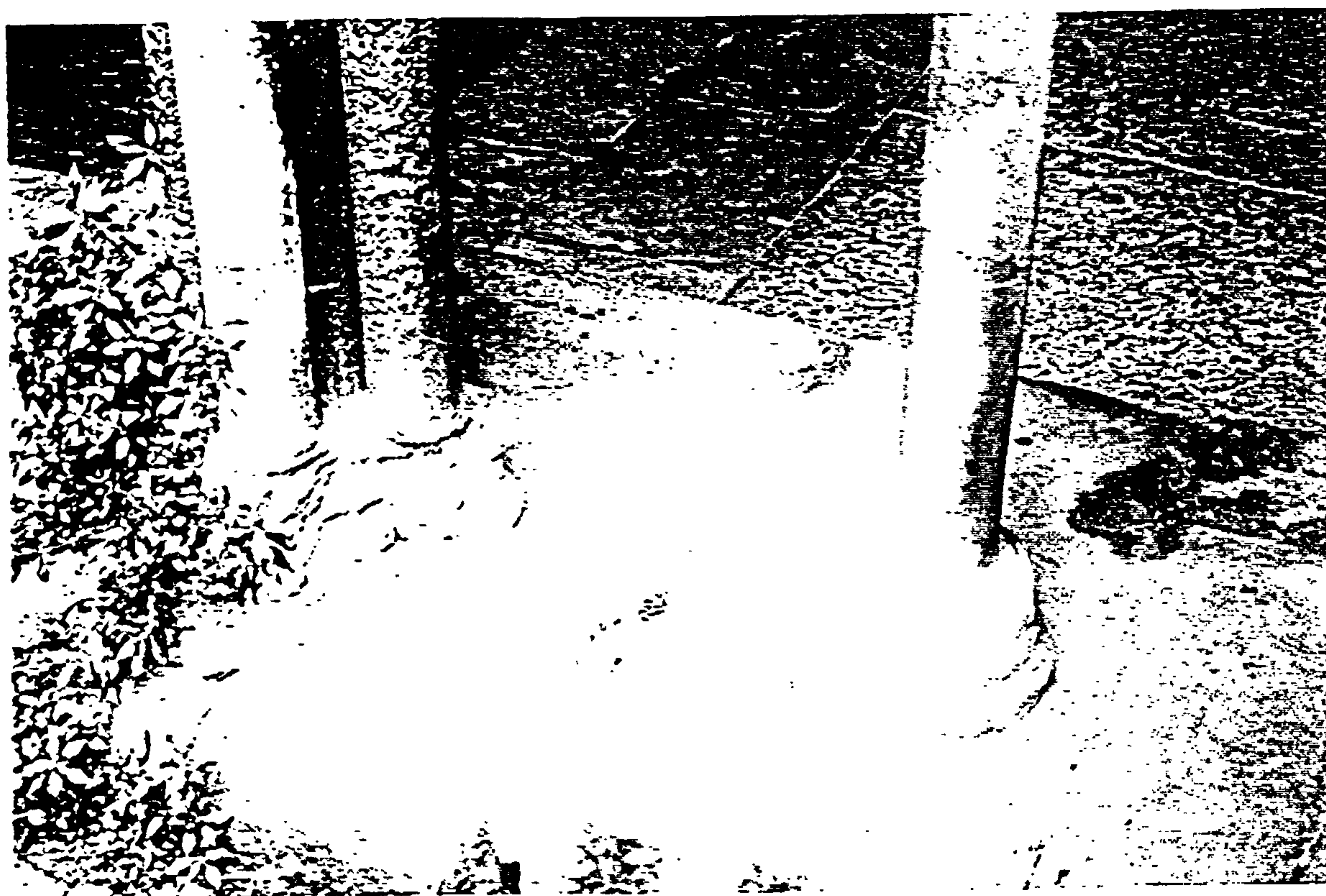
Plate 1.9 Eroded pillars, Salisbury cloisters
