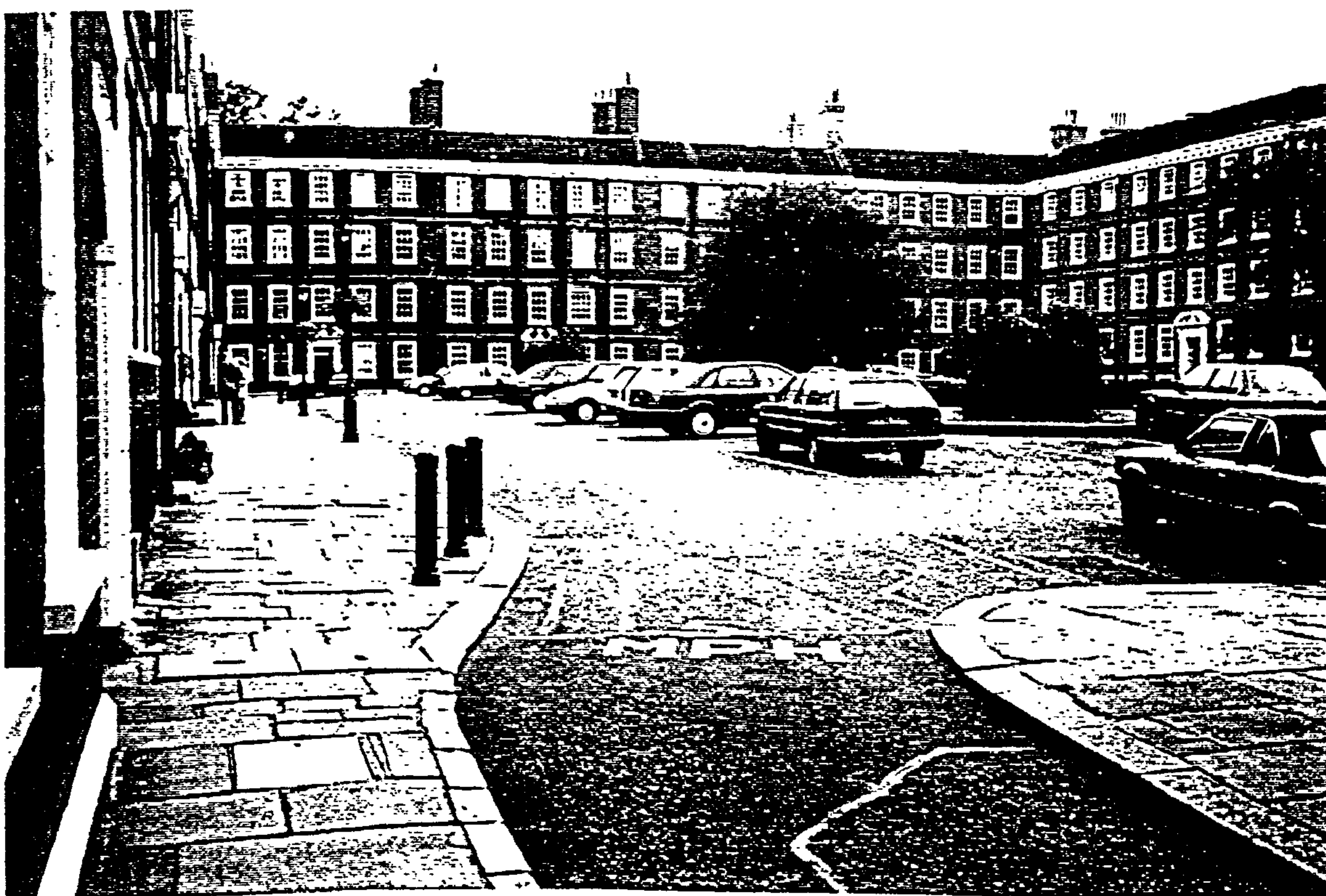
Plate 4.4 Paving, kerb and guard posts, Grays Inn
