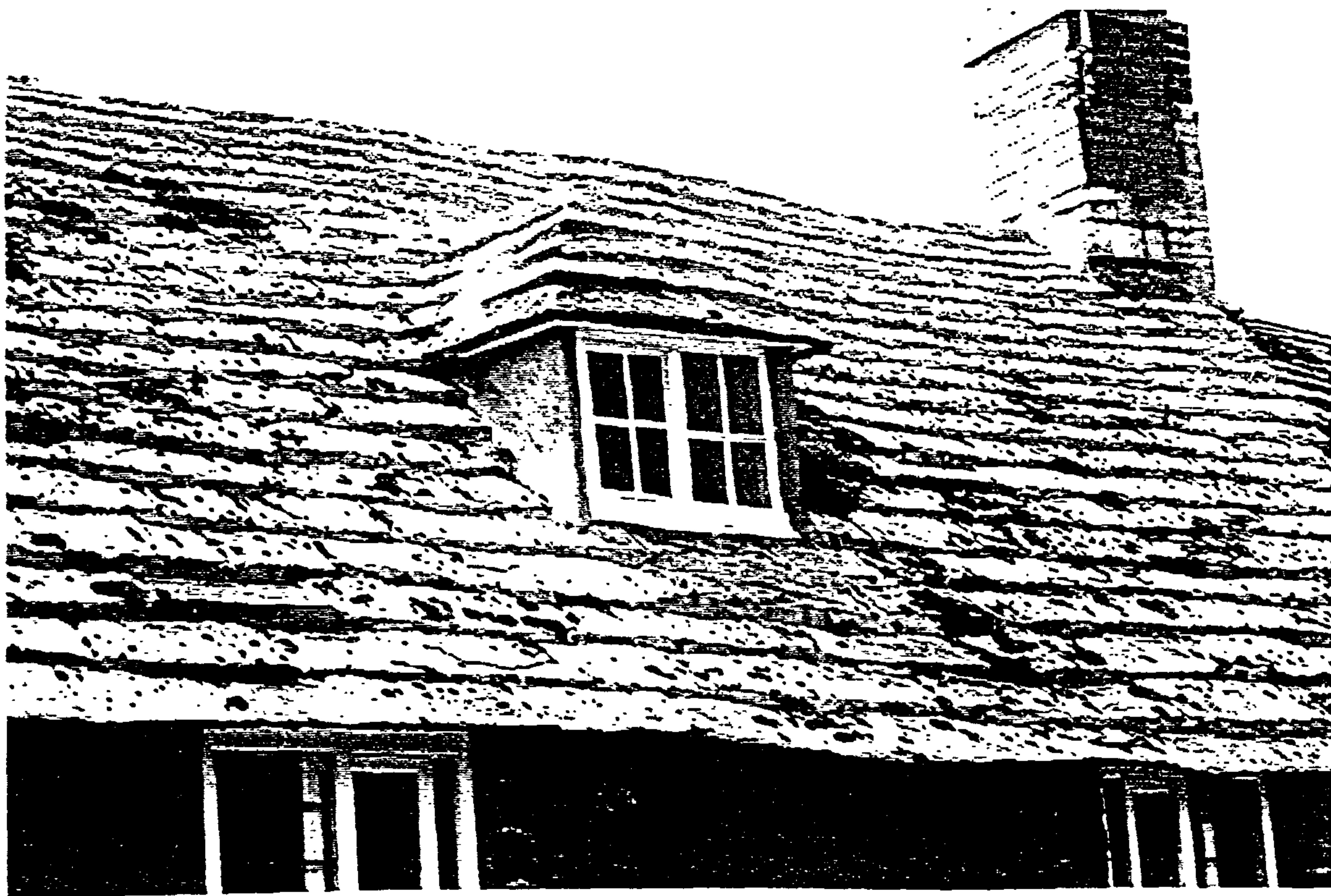
Plate 11.4 Mortar flushing of tiled roof, Corfe Castle
