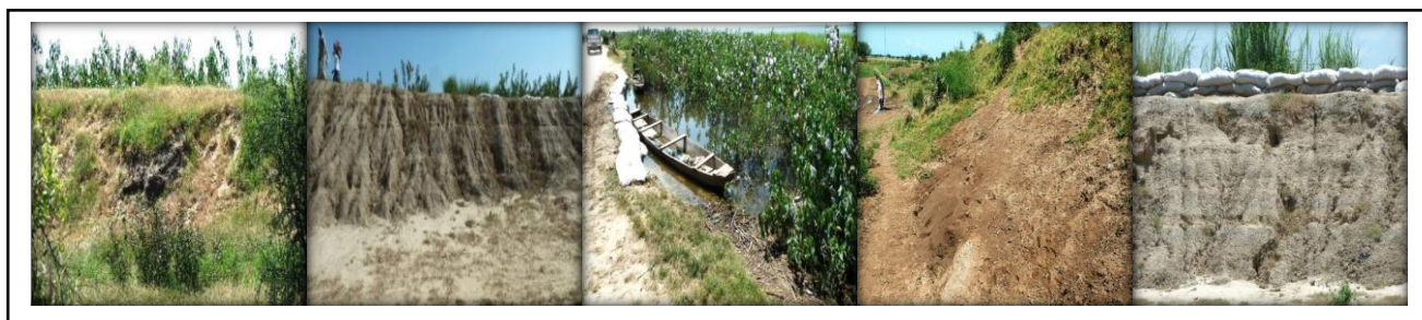
Figure 7. Pictures showing deterioration of the Maga Dam
