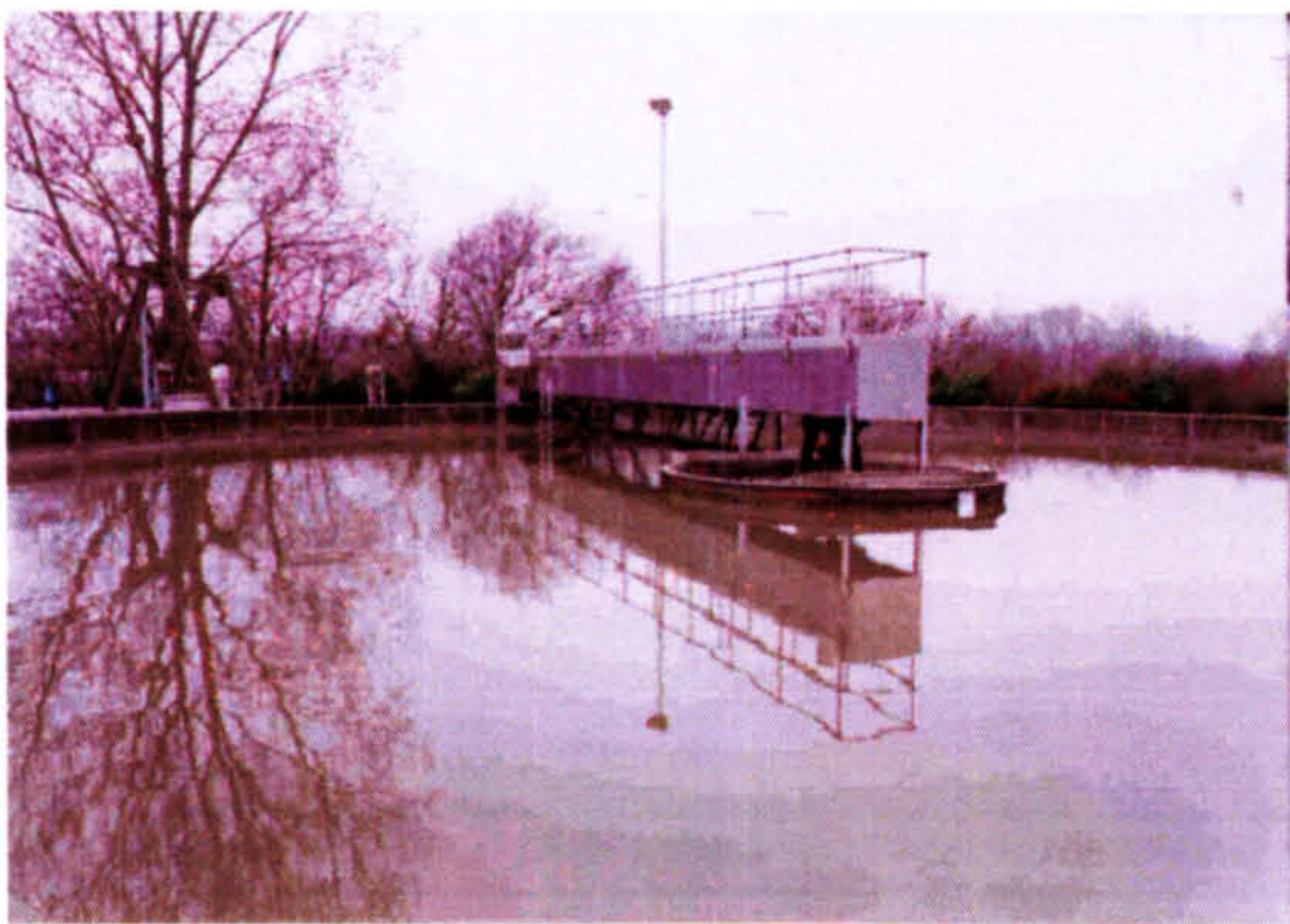
Figure 1.2b. Wastewater in a settlement Tank; the first stage of treatment.
