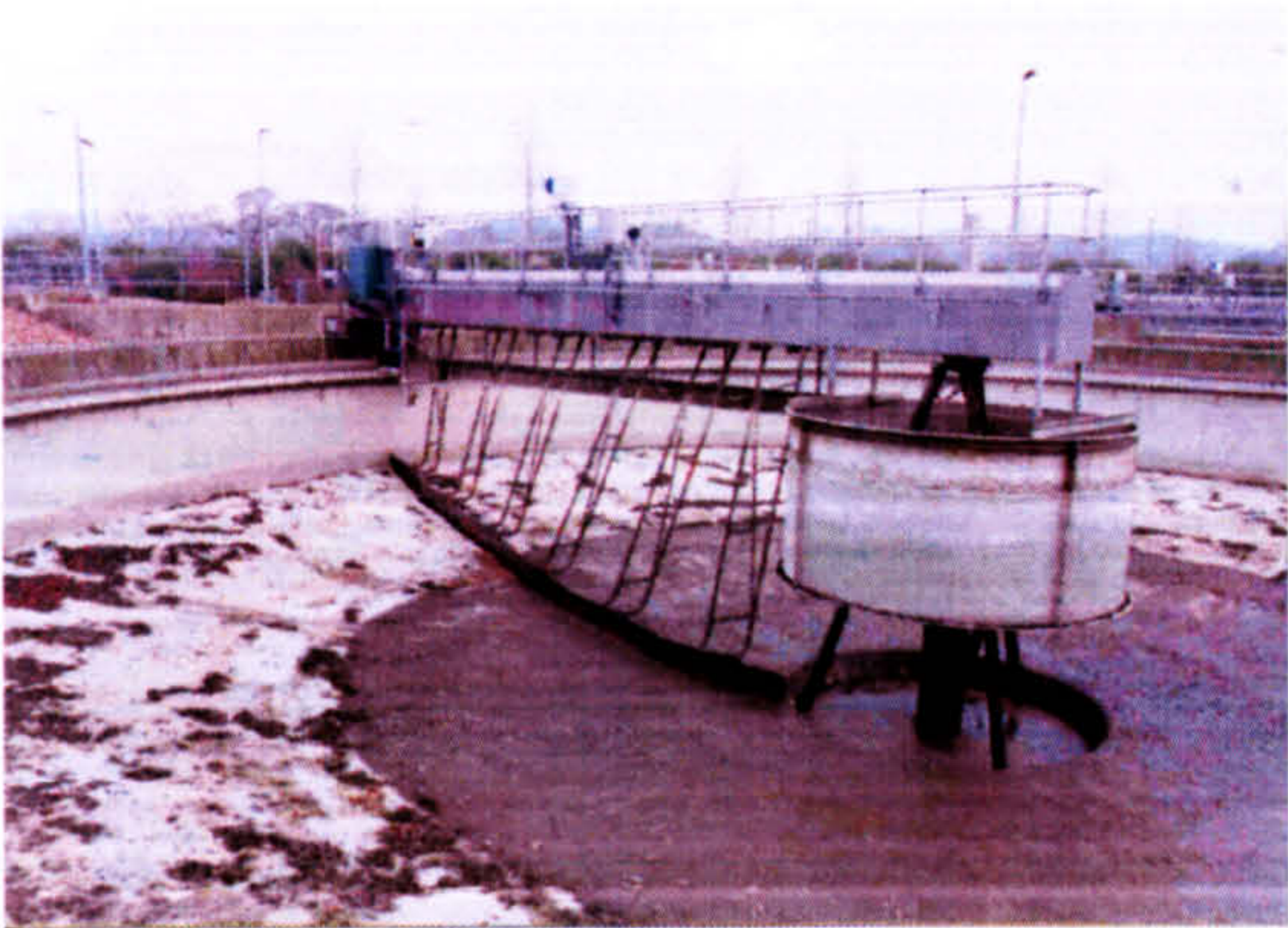
Figure 1.2c. The solid phase settles to the bottom of the tank and is pumped to a sludge digestion plant.
