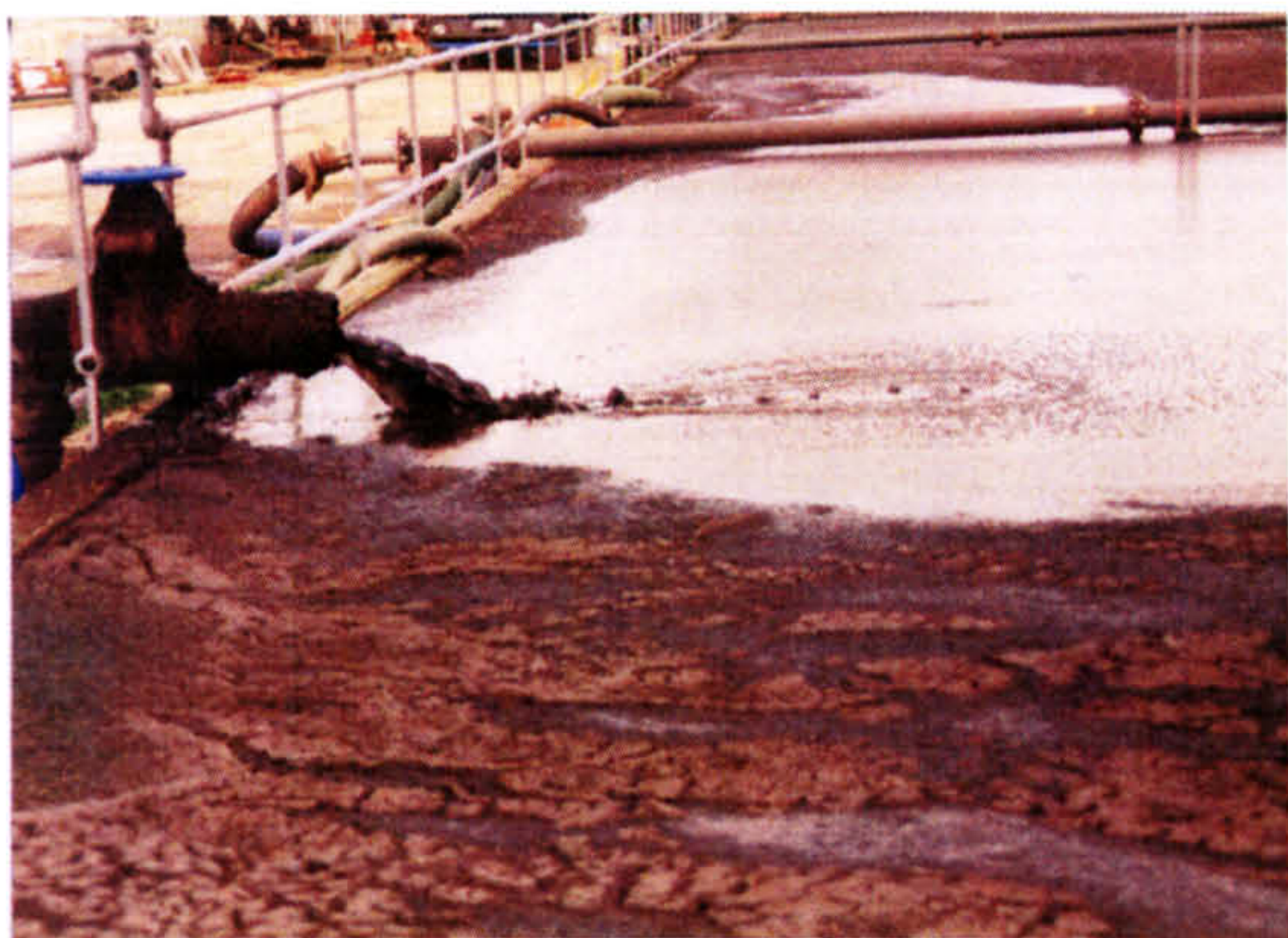
Figure 1.2e. Sewage sludge entering a drying lagoon. The digested sludge leaves the digester with a dry matter content of ca 5 %. This may be injected directly into agricultural soil or the dry matter content can be increased to ca 20 % in lagoons to form a sludge ‘cake’
