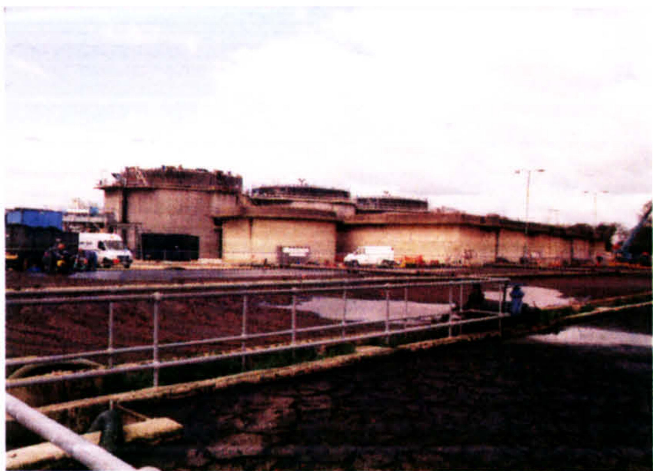
Figure 1.2d. An anaerobic sludge digestion plant looking across the drying lagoons. The volume of sludge is reduced by 70% in the digestion process.
