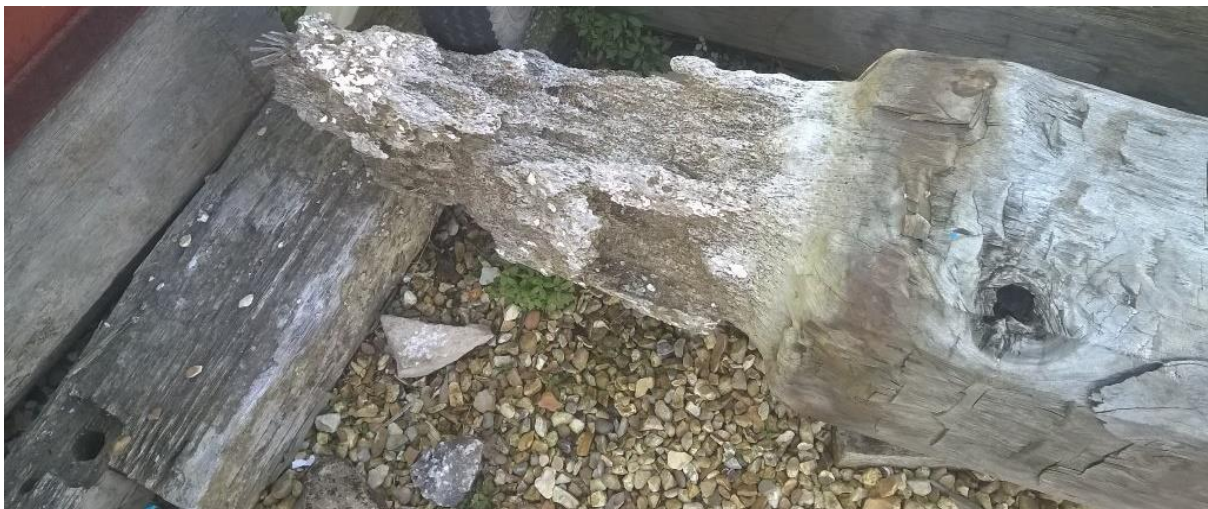
Damage caused by gribble worms to one of the wooden piles at Swanage Pier (Source: Anya Chapman)
