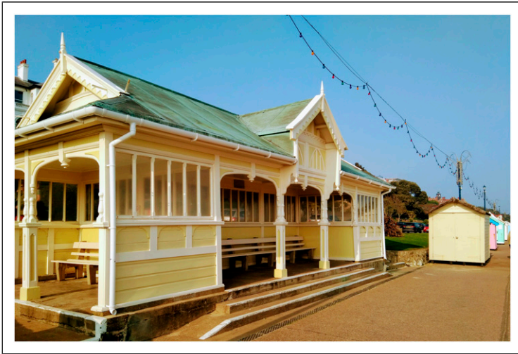
Figure 3. Shelter at Felixstowe.
