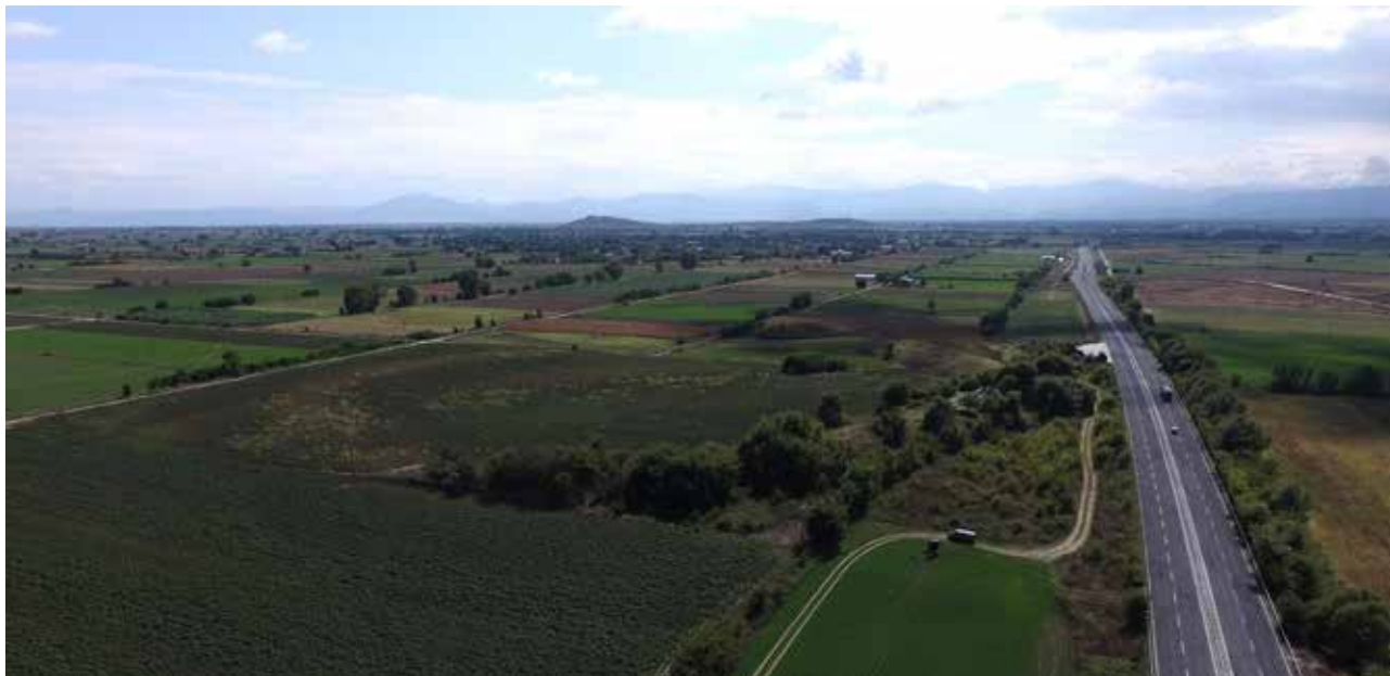
Fig. 14. Aerial view of the Chomatokastro site, looking towards the south. At the horizon is the acropolis of ancient Kierion. Photograph by Derek Pitman.
