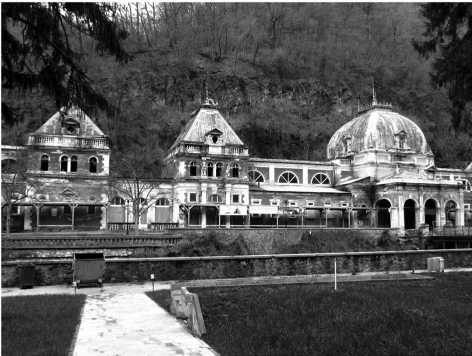
Figure 1. Derelict building in Băile Herculane (courtesy of Ana Ianas).
