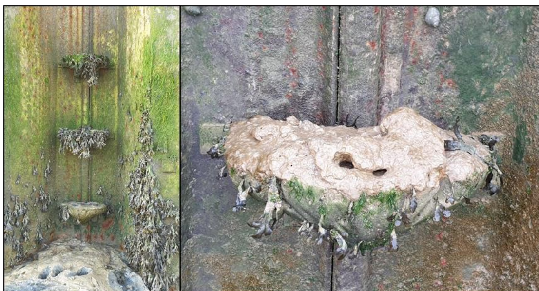
Figure 38. Left: One of the three columns of artificial rockpools. The rockpools were fixed to the in-pan of the steel sheet piling. The top rockpool was fixed at approximately Mean High Water Neap Tide Level. The foot of the sheet piling was approximately Mean Tide Level. Right: an artificial rockpool on the steel sheet piling filled with mud, photographed 2.5 years after installation.
