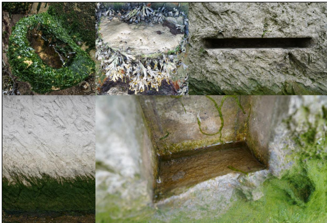
Figure 2. Examples of coastal eco-engineering. Top left, clockwise: An artificial rockpool containing water (Marineff Project); a Vertipool containing mud (Bone et al. 2022); a 'letter box' crevice in a concrete seawall; a cubic void containing water in a concrete seawall; a concrete seawall with a 'rockface' textured surface created with a formliner. Images by Jessica Bone.
